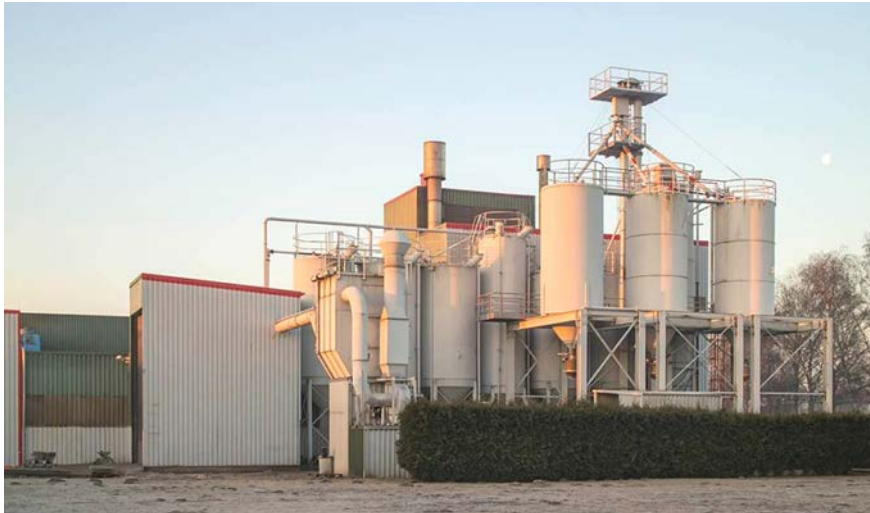
Fig. 1 Used and reclaimed sand offloading silo at the HA works in Braunschweig.
